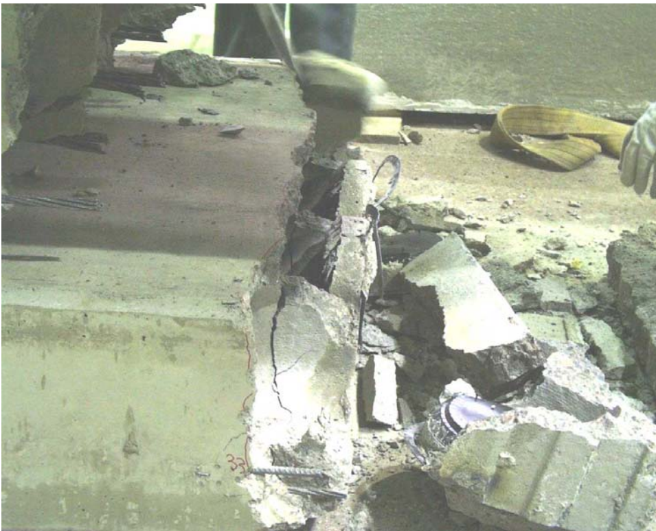
Fig. 20. End of western slab.
