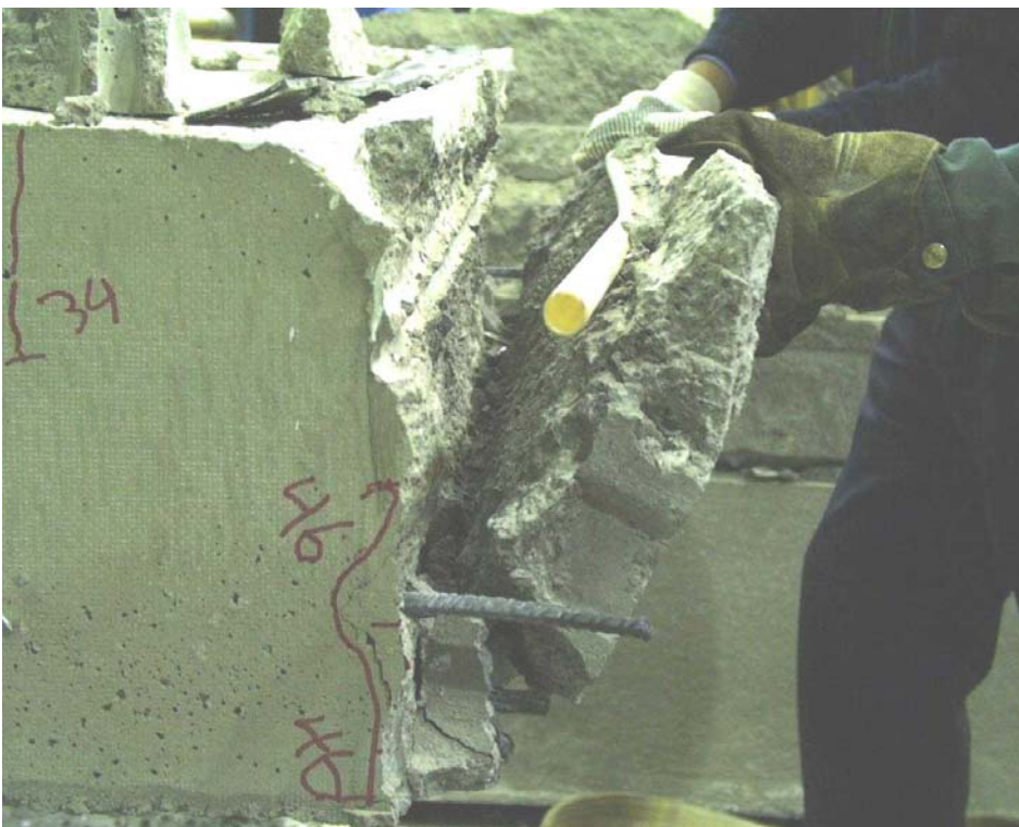
Fig. 22. Removing a concrete block from end of western slab.
