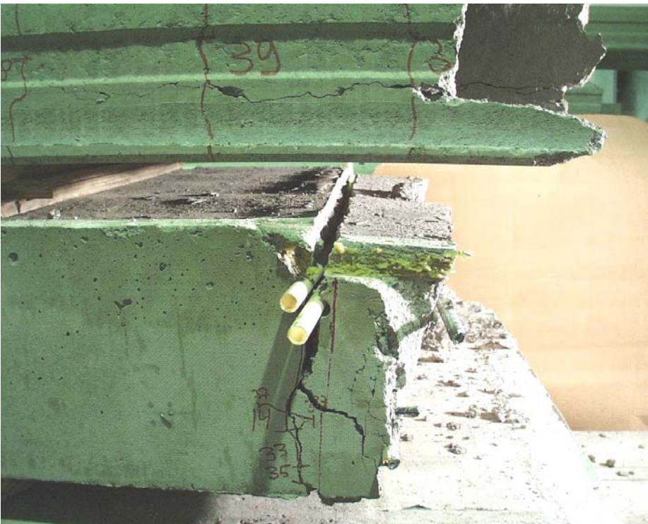
Fig. 20. End of eastern slab.
