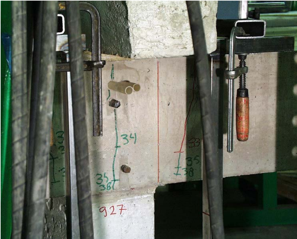
Fig. 7. Cracks at step 38 seen from north.
