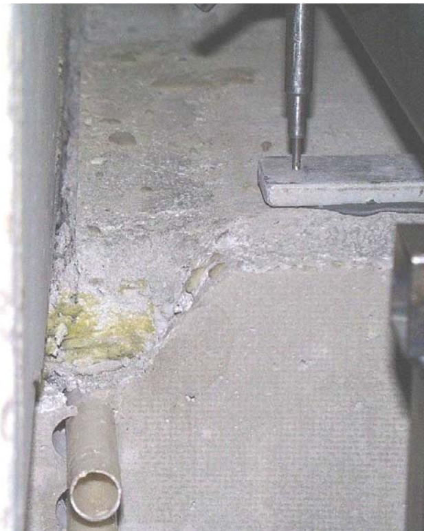
Fig. 10. No visible cracking in upper wall element after failure, seen from east.
