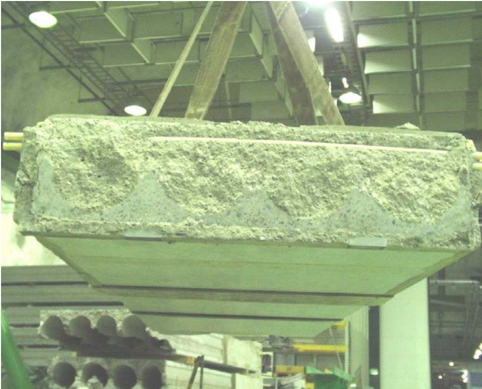
Fig. 15. End of western slab.
