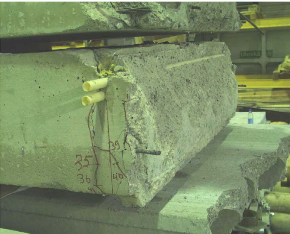
Fig. 22. End of western slab.
