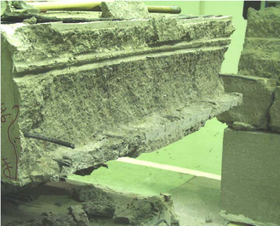
Fig. 23. End of western slab.
