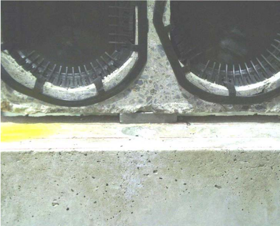
Fig. 1. Steel plate under hollow core slab.
