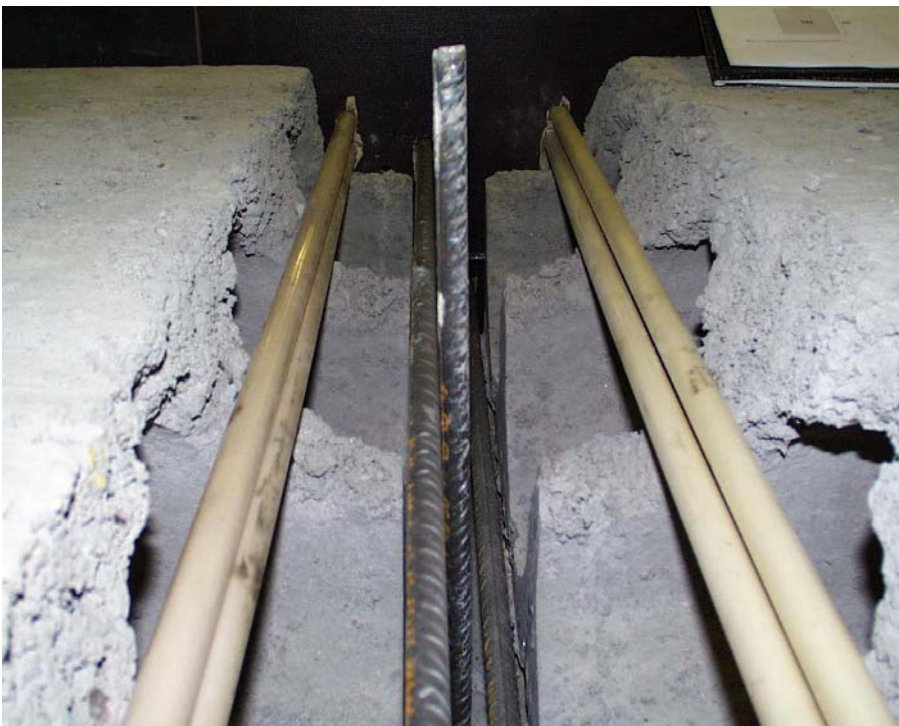
Fig. 2. Joint before concreting.
