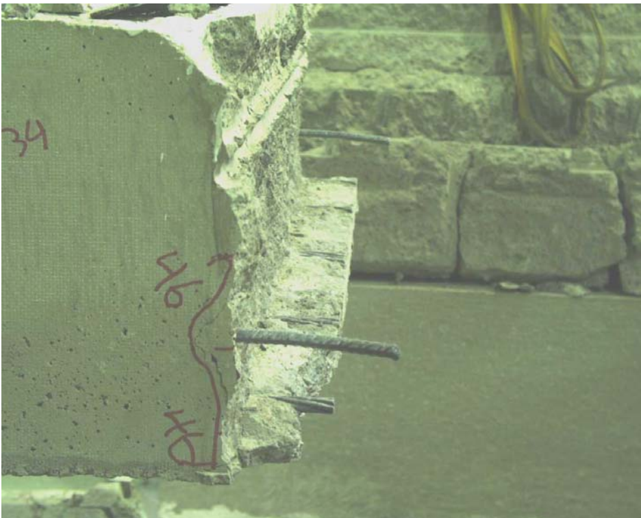
Fig. 24. End of western slab.
