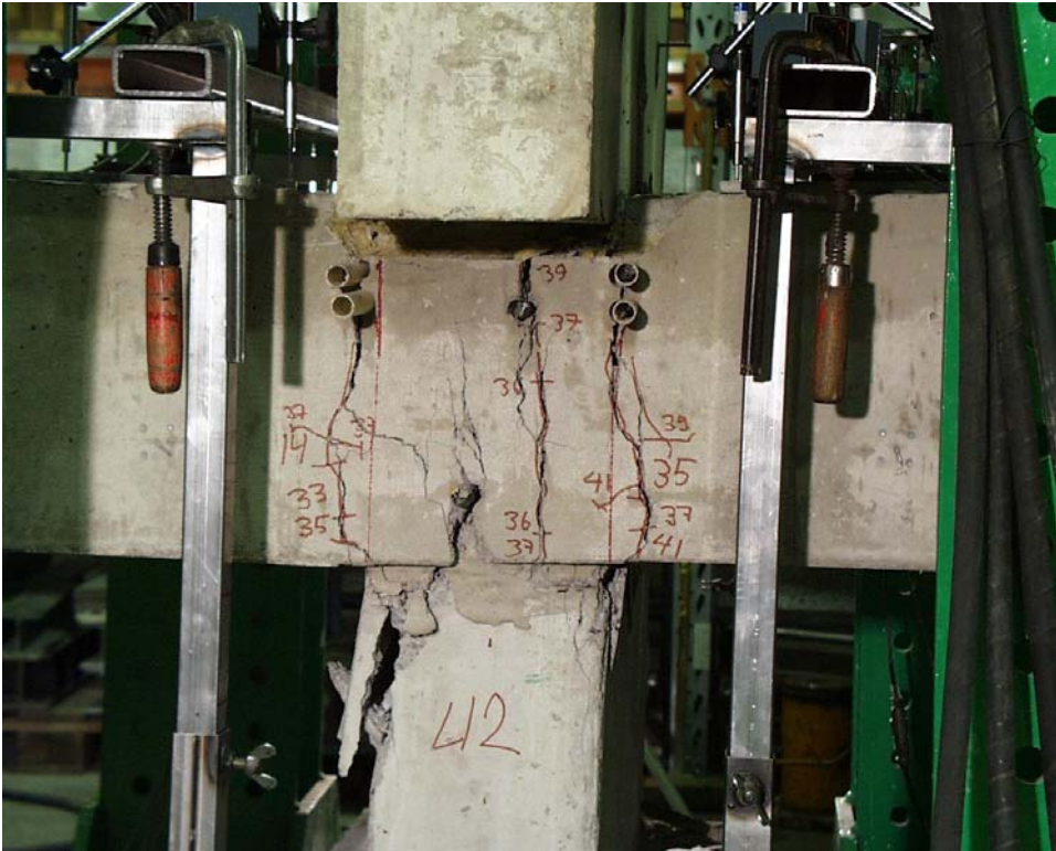
Fig. 3. Cracking pattern at failure seen from north.
