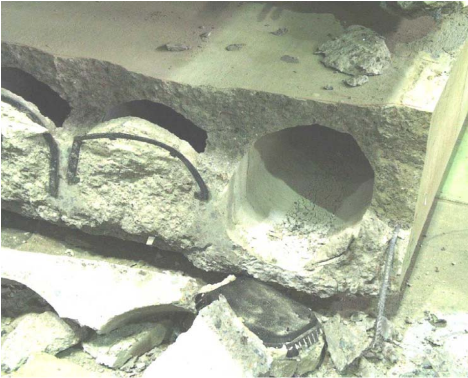
Fig. 21. End of western slab.
