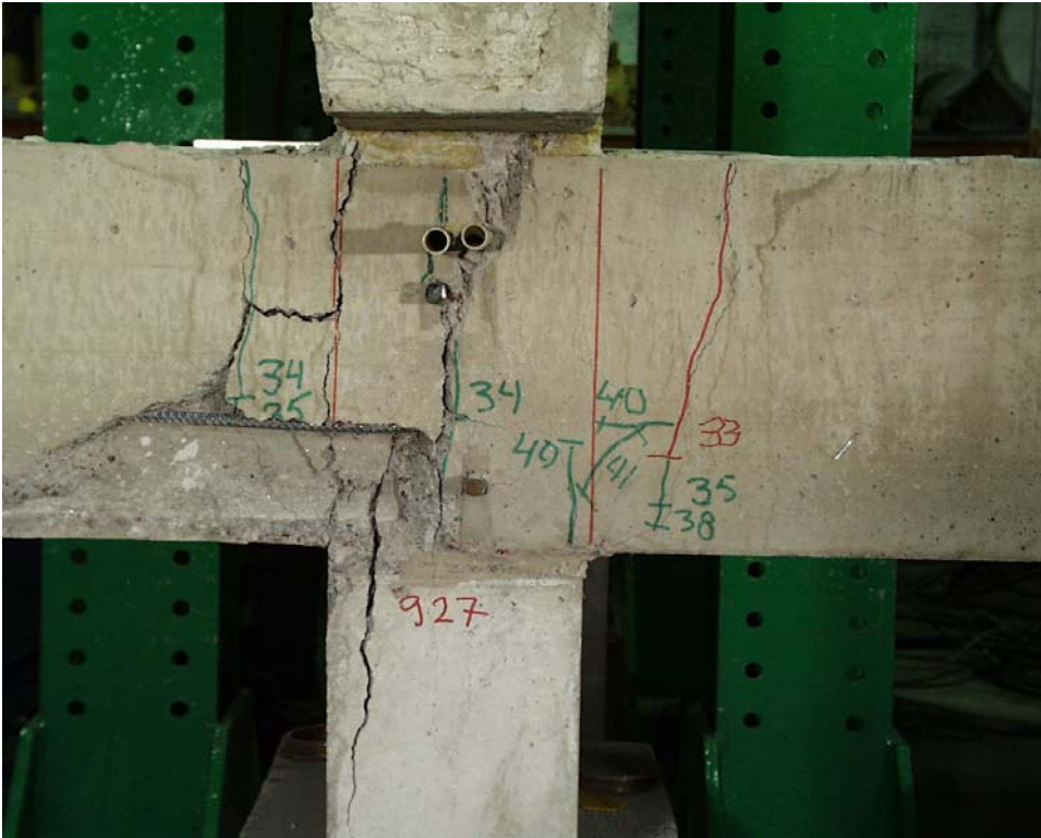
Fig. 11. Cracking pattern after failure seen from north.
