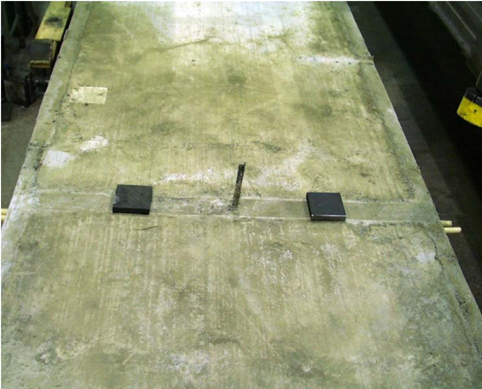
Fig. 3. Steel plates to support the upper wall element.
