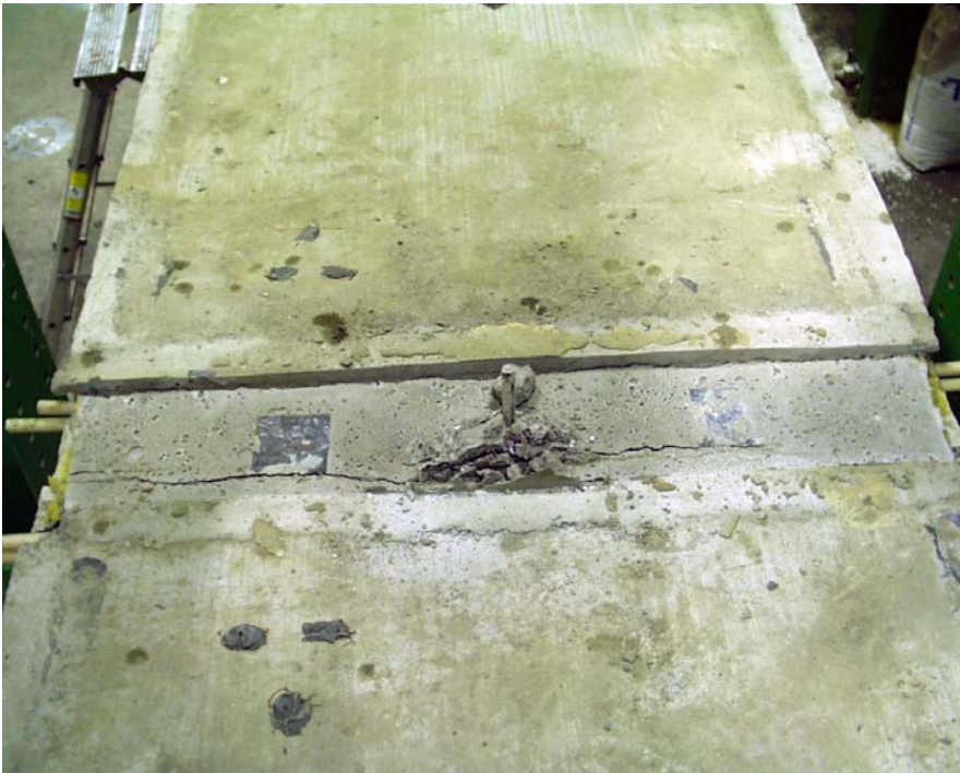
Fig. 12. Joint after removal of the upper wall element seen from west.
