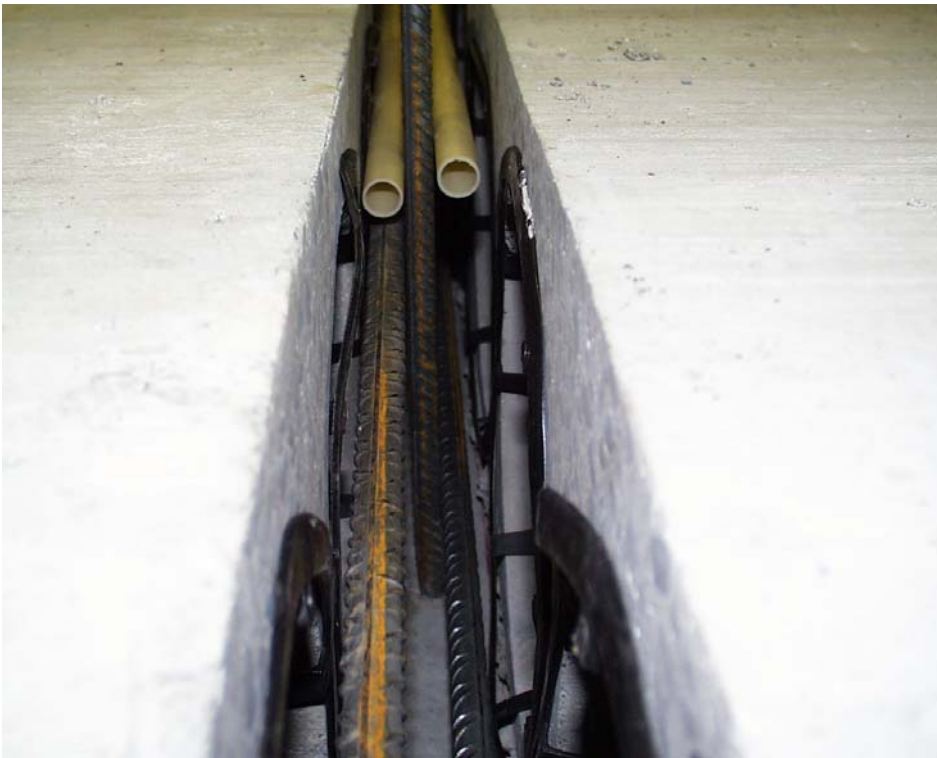
Fig. 2. Joint reinforcement and plastic pipes being pushed to their final position .
