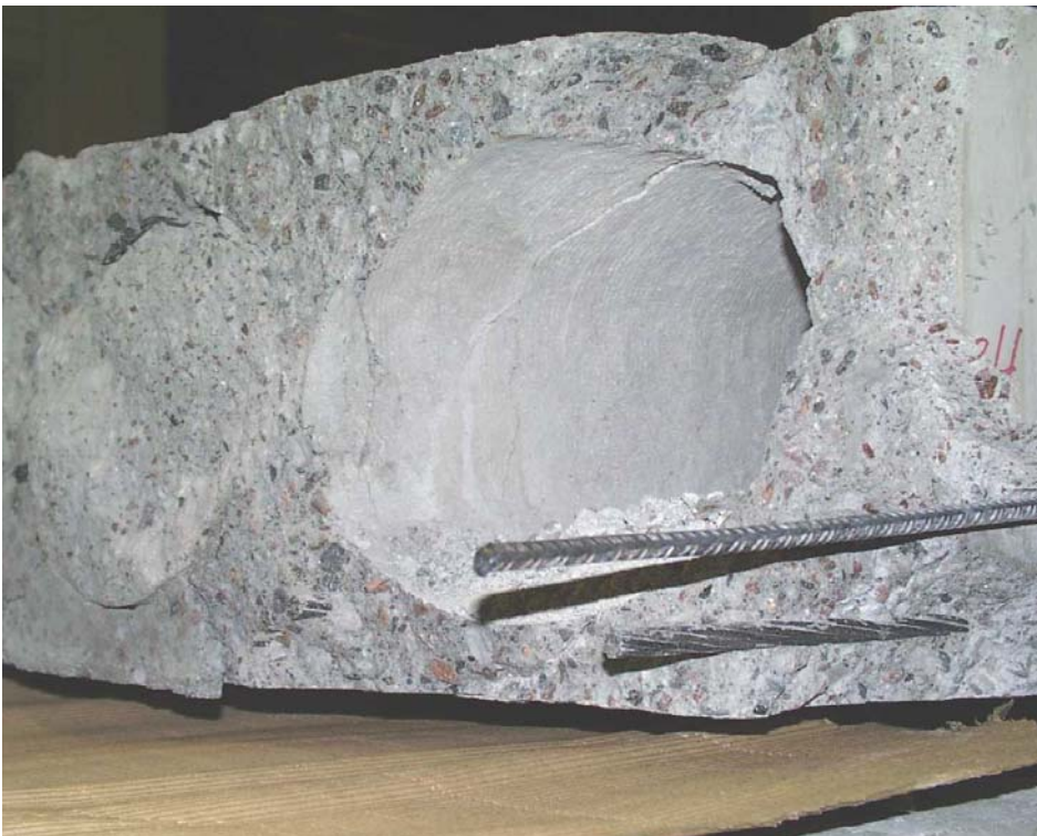
Fig. 22. End of eastern slab.
