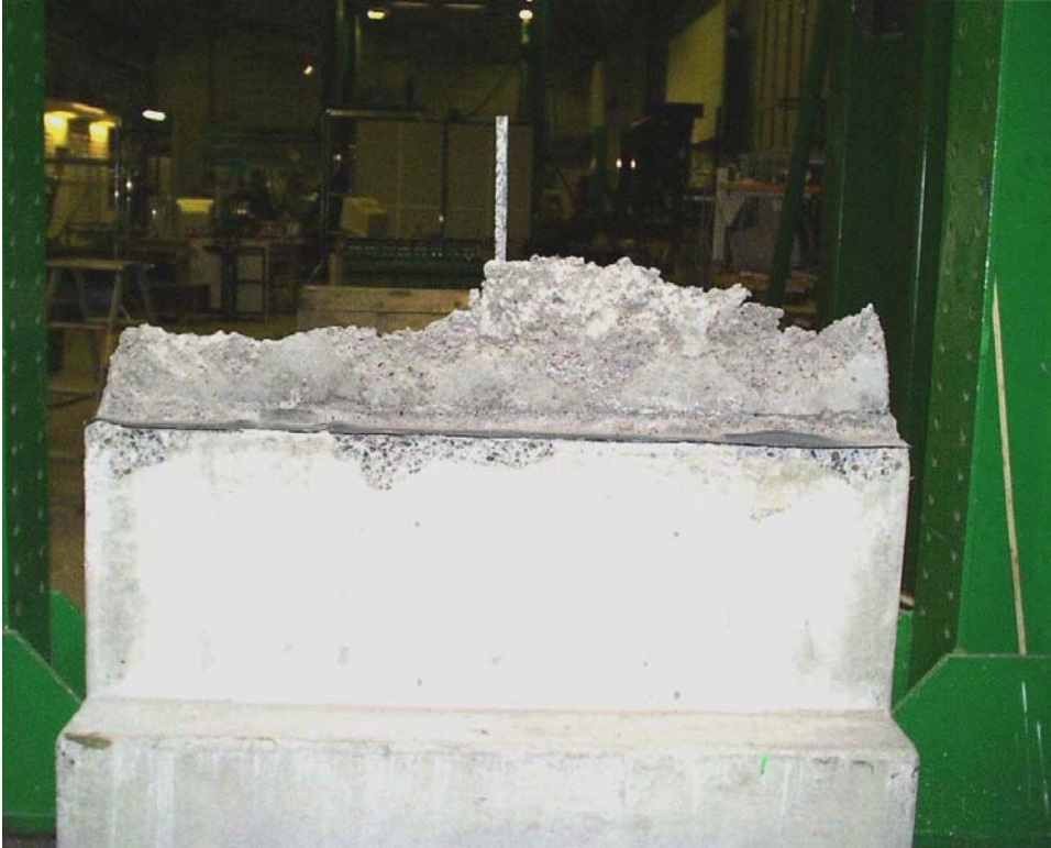
Fig. 17. Lower wall element seen from west.
