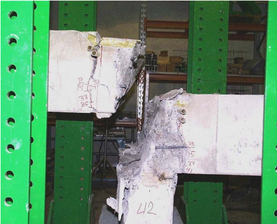
Fig. 13. Removal of the failed slab seen from north.
