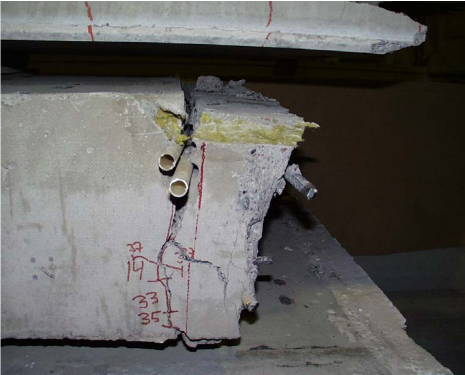
Fig. 19. End of eastern slab.
