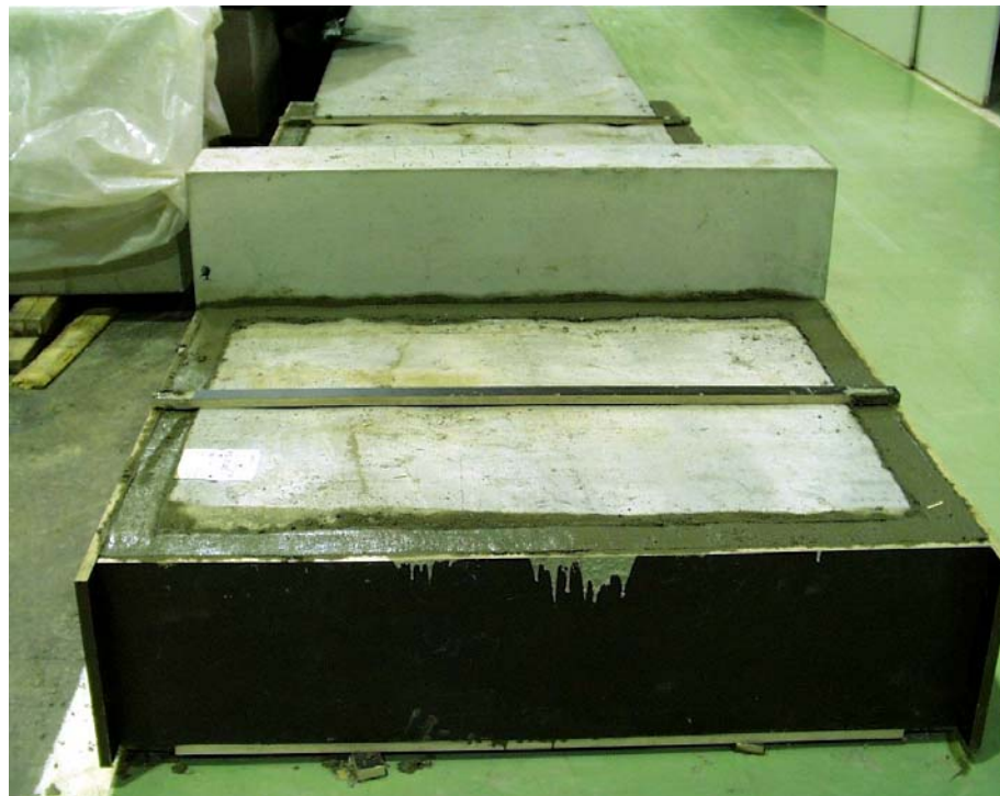
Fig. 6. NI. Grouting completed.
