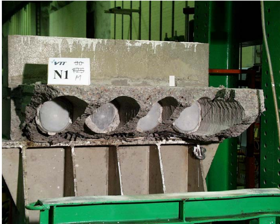
Fig. 21. N1. Joint after removing main part of slab element
