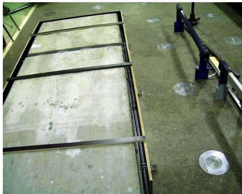
Fig. 2. Edge of slab before grouting.
