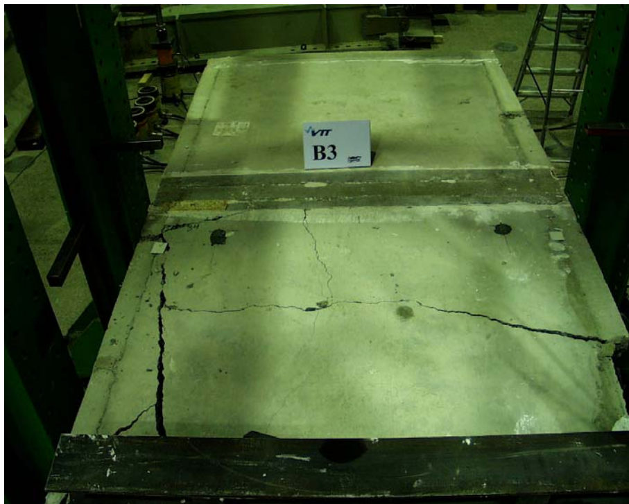
Fig. 44. B3. Top surface after failure.
