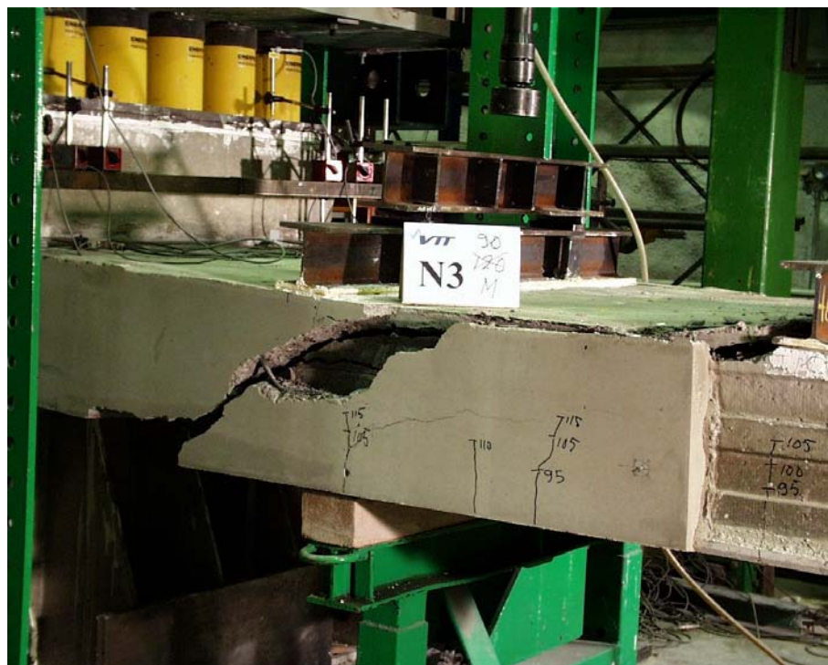
Fig. 40. N3, North edge. Failure crack and flexural cracks.
