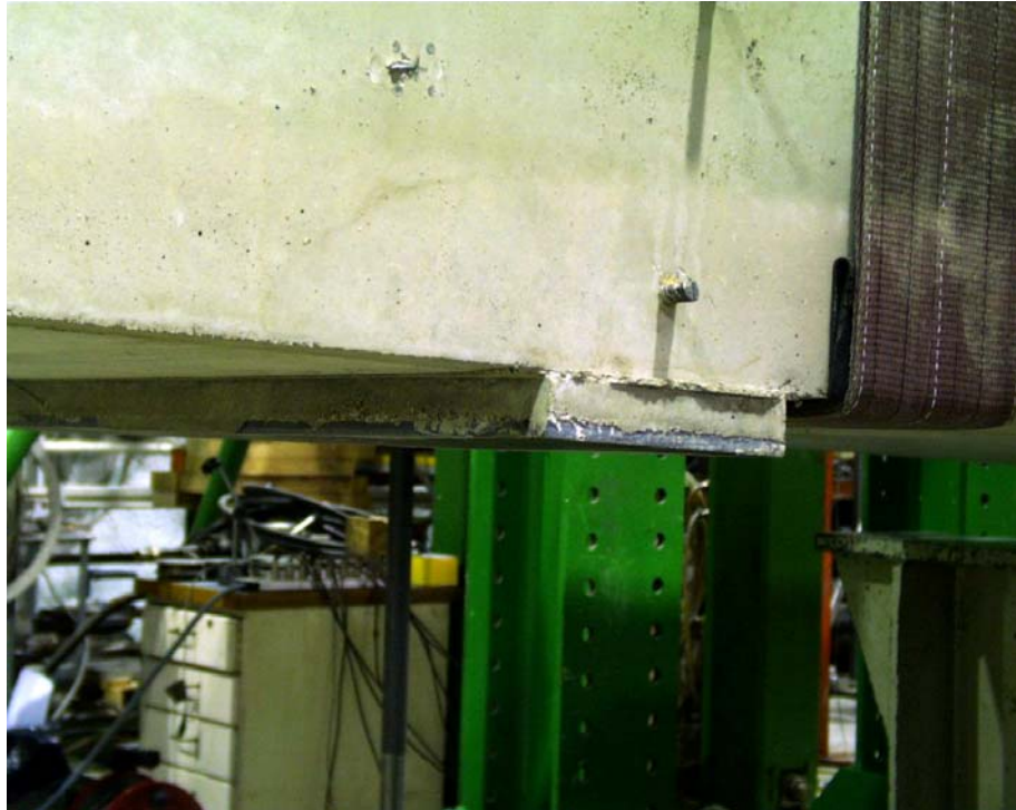
Fig. 5. Steel plate and mortar below jointed slab ends .
