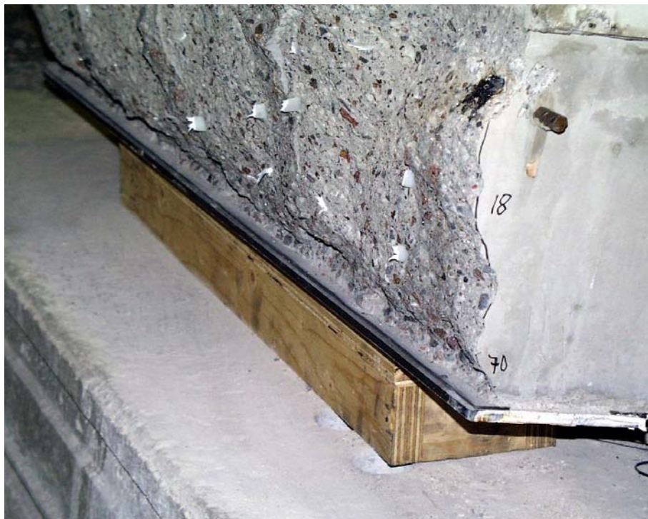
Fig. 36. N2. Flexural crack.
