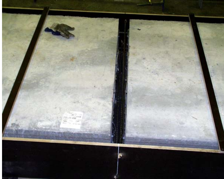
Fig. 1. Joint before grouting.
