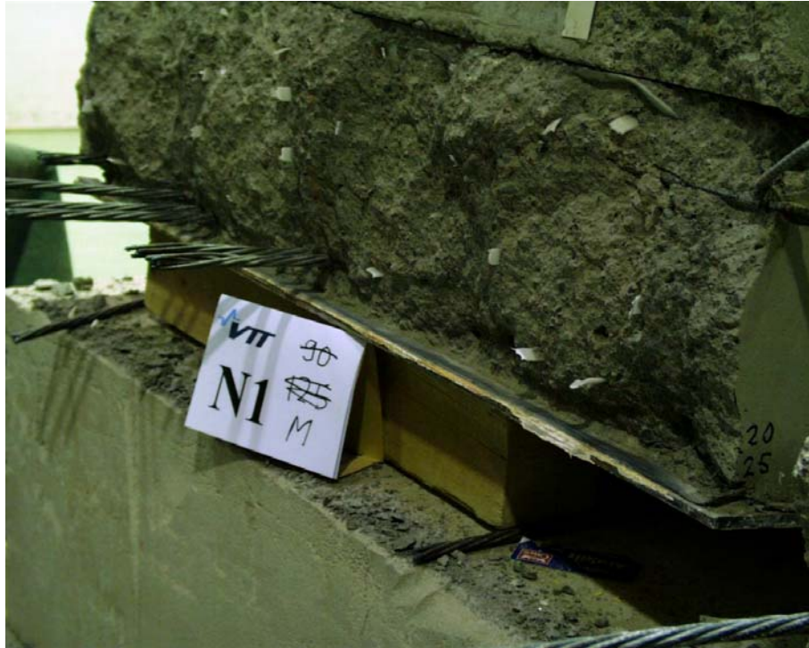
Fig. 23. N1. Vertical crack.
