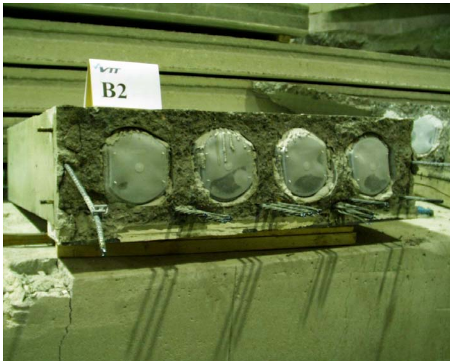
Fig. 34. B2. Flexural crack after flame cutting the strands and the tie bars.
