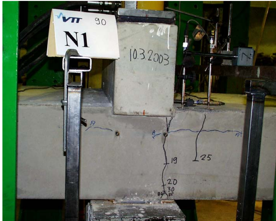
Fig. 9. N1, North edge. First cracks.
