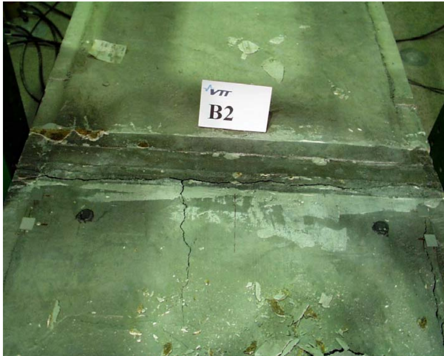
Fig. 33. B2. Top surface after failure.
