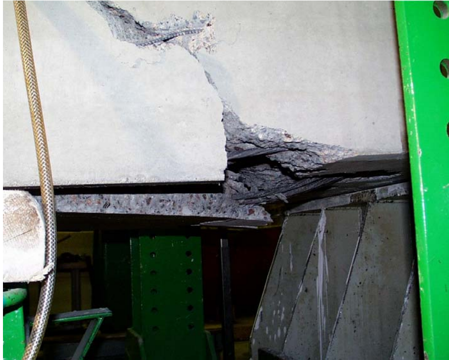
Fig. 43. N3, South edge. Failure crack.
