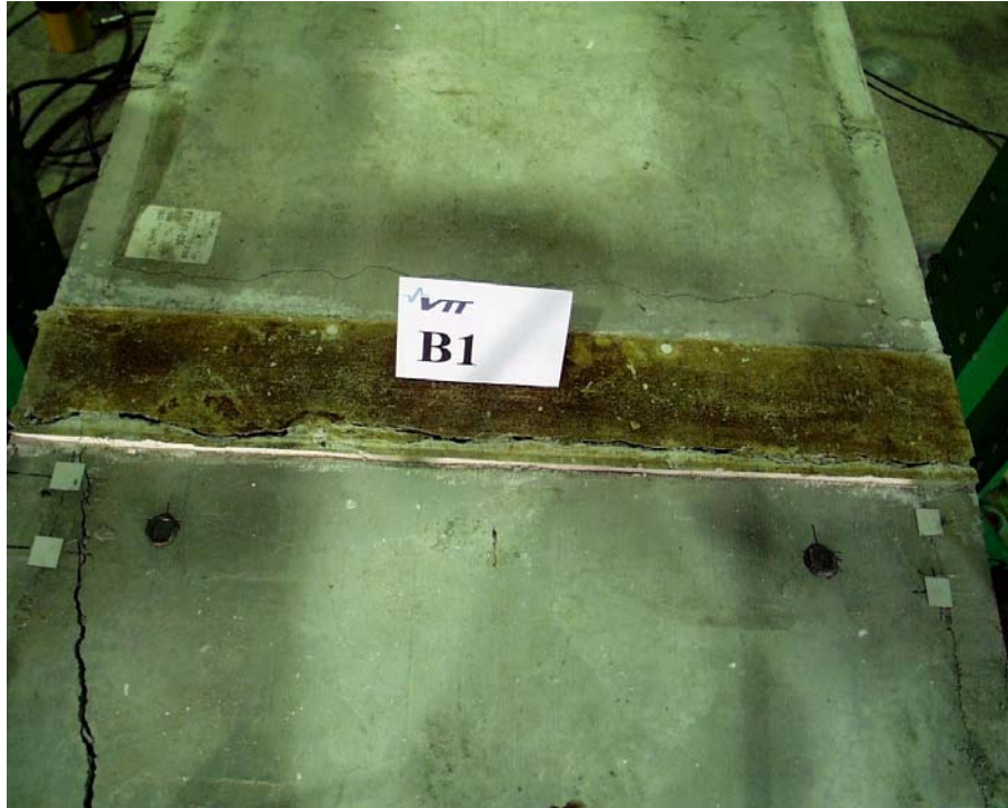
Fig. 19. B1.III. Top surface after failure.
