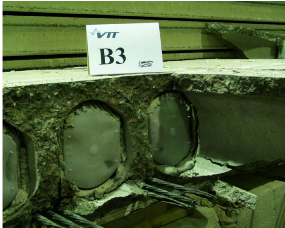
Fig. 49. B3. Detail of flexural crack.
