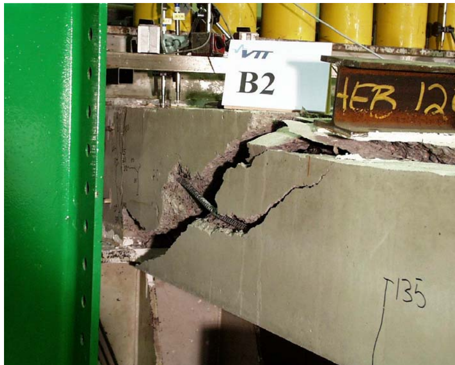
Fig. 28. B2. North edge after failure.
