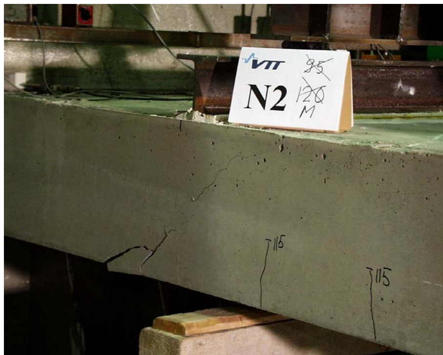
Fig. 26. N2, North edge. Failure crack and flexural cracks.
