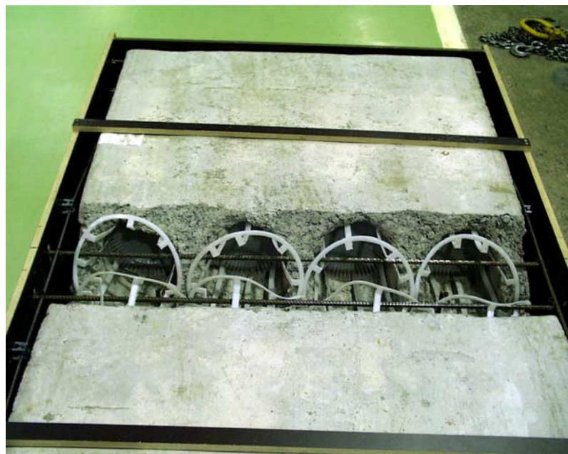
Fig. 2. N1. Joint before grouting.
