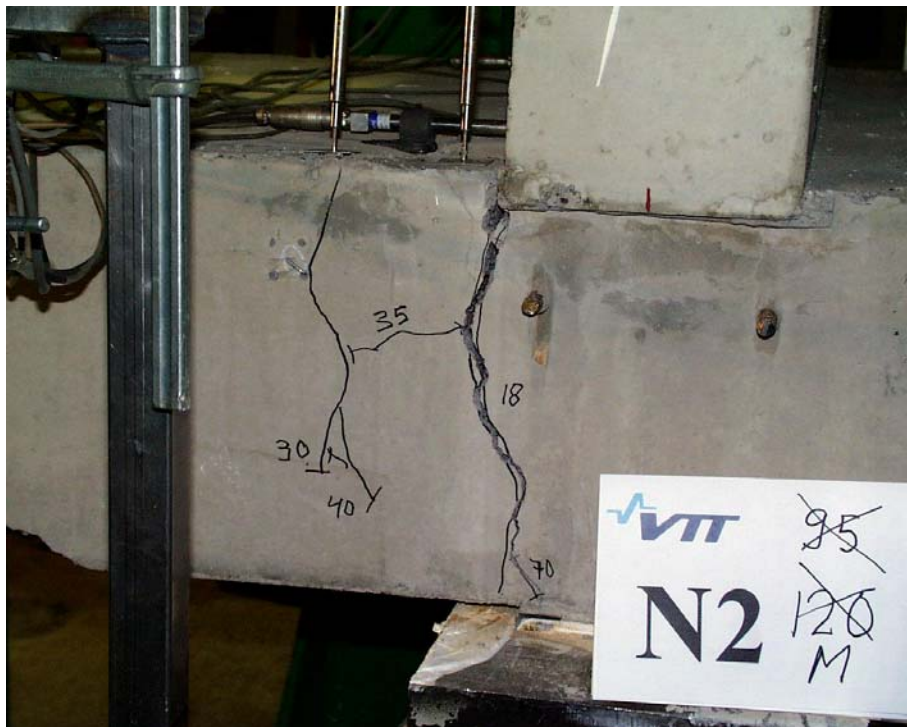
Fig. 30. N2, South edge. Cracks next to the joint after failure.
