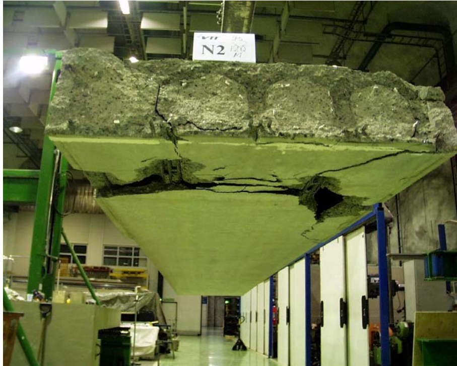
Fig. 37. N2. Soffit and cracked end of slab.
