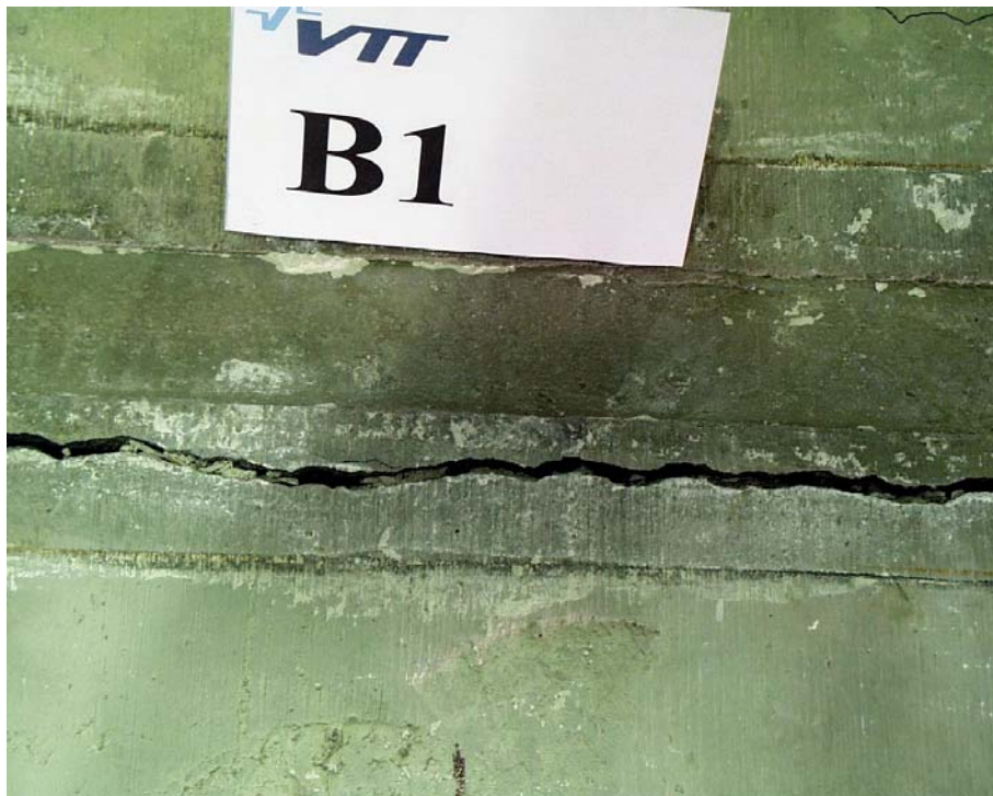
Fig. 20. B1.III. Top surface after failure. Note that the slab end is cracked, not the joint concrete.
