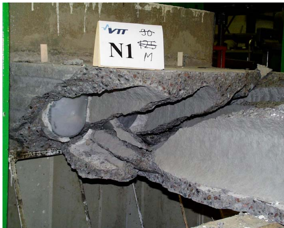
Fig. 20. N1. North edge after removing a loose corner of slab.
